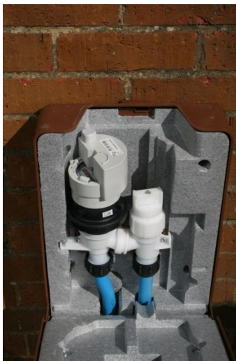
Groundbreaker with Sensus Meter and "Water Spy"
